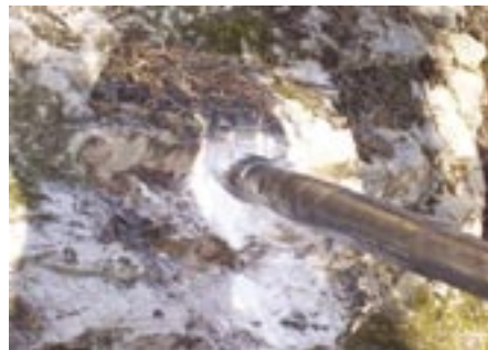
Starting the cable-guided pilot bore
