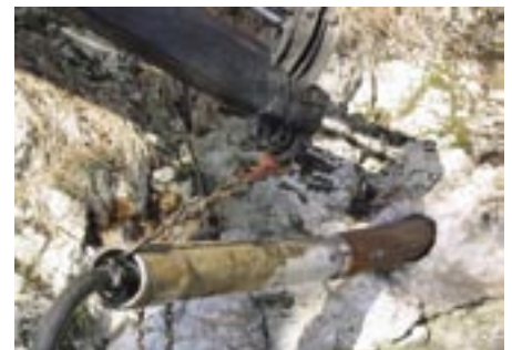
The Olymp ramming the steel pipes
