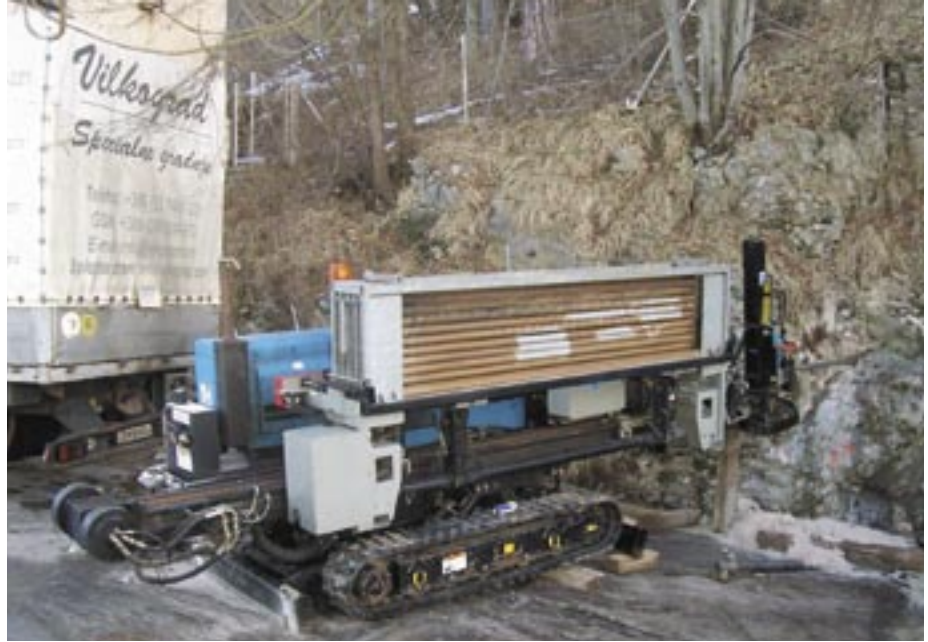
Grundodrill bore rig during the pilot bore
